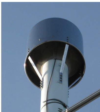
Fig. 3-3b: (b) New-design sampling stack rain cap.
