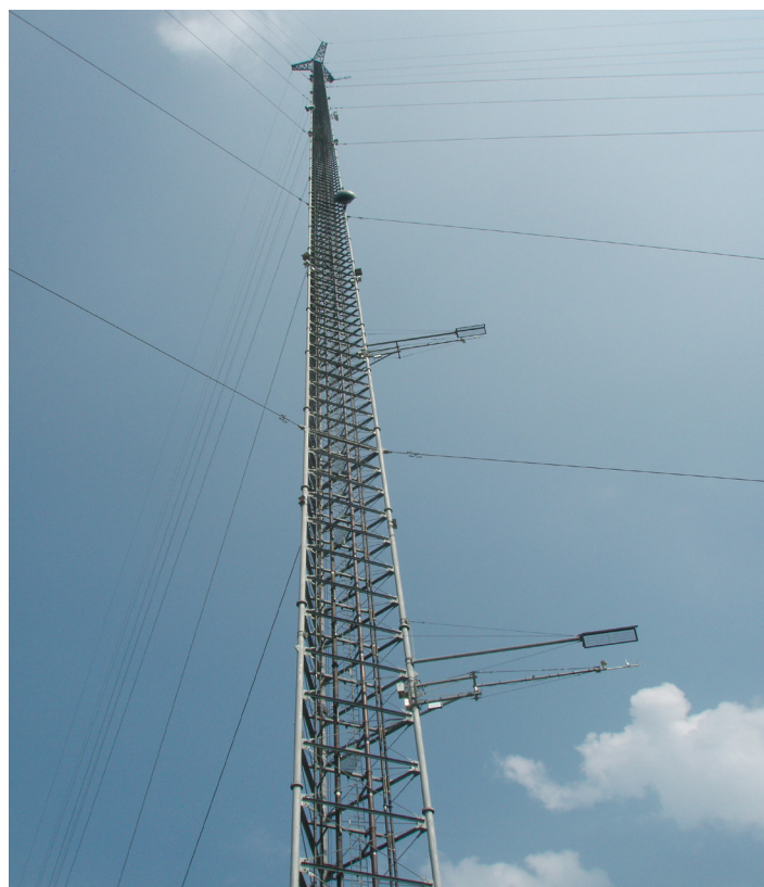
Fig. 4-6: Tall tower at Beech Island, South Carolina. Air sampling intakes at 30, 61, and 305 m above ground.
