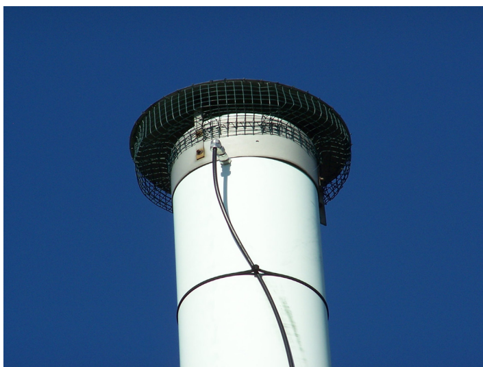
Fig. 3-3a: (a) Old-design sampling stack rain cap.
